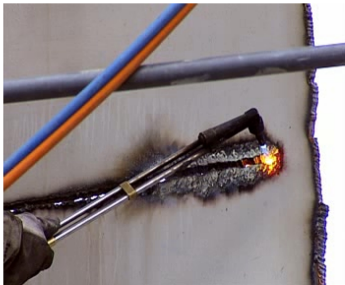
Fig.15 – Taglio del liner interno dell’impianto di Kahl (fonte: “The Kahl nuclear power test plant – Dismantling the reactor building”, NUKEM GmbH)
